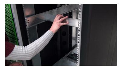
Figure 1-15 Slide the Alignment Tool from Front to Back
