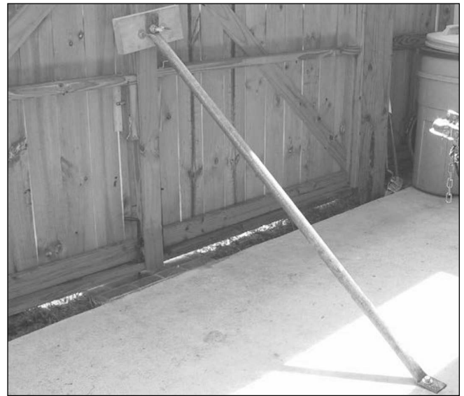
A suitable length of heavy-wall pipe is anchored to the gate at one end and the concrete pad at the other. This considerably increases the wind resistance of the gate.
