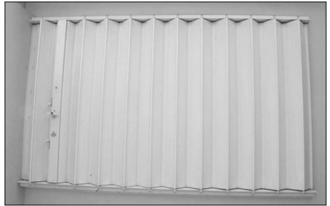
Accordion type hurricane window shutters can be closed and latched in just seconds.
