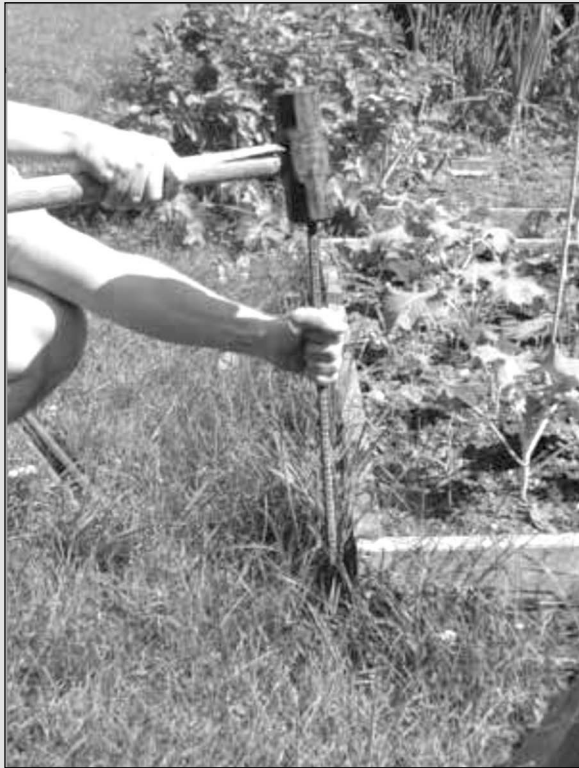
Driving the rebar into the ground
