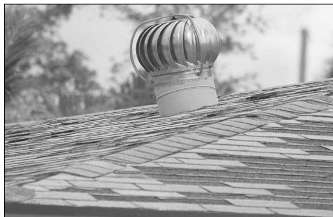
Wind turbines like this one should be removed and the opening capped before the storm arrives.
