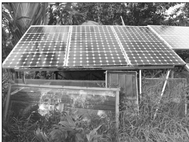
A solar panel with individual cells visible. The cells convert the sun's energy into electricity when sunlight falls on a special layer of silicon and makes electrons move, creating a potential difference between layers. In this picture, lying below the solar panel array are a couple of old solar collectors.
