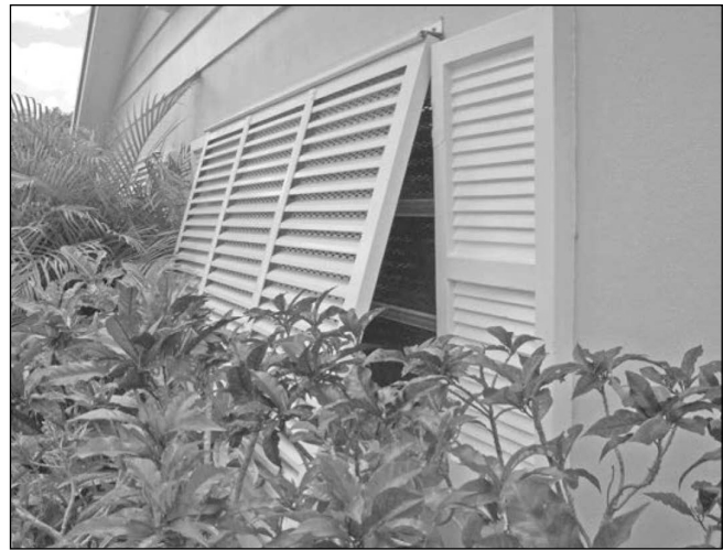
Hurricane-proof aluminum Bahama shutters can be lowered to completely cover the window.
