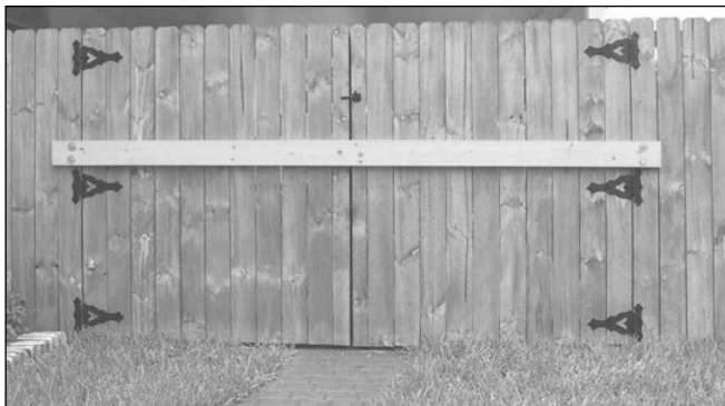
A 2x8 is used as a brace to strengthen this double gate.
