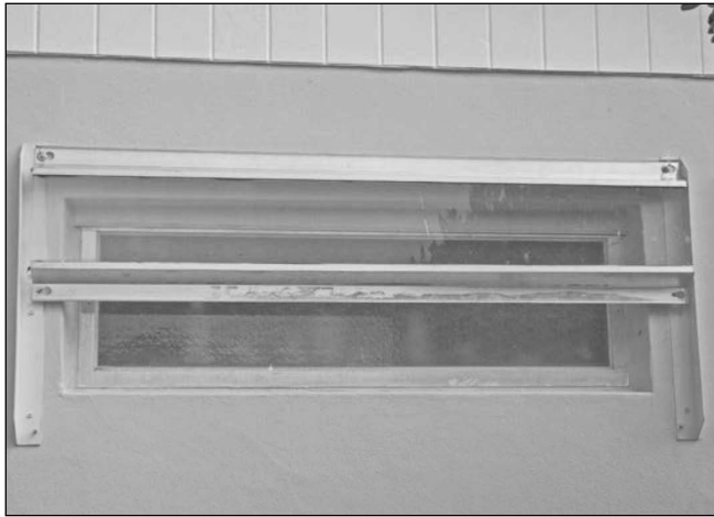
These vertical tracks allow storm panels to be mounted horizontally. Note the top panel is mostly clear to allow light in.
