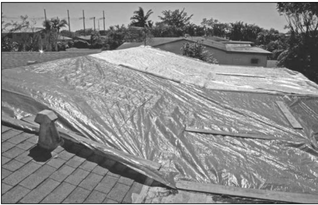
Blue and silver plastic tarps used to cover a hurricane-damaged roof
