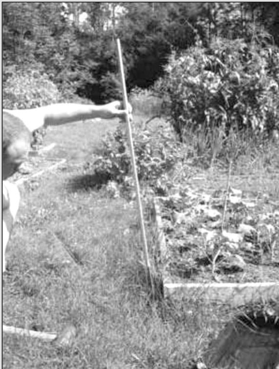
Placing an upright over the rebar
