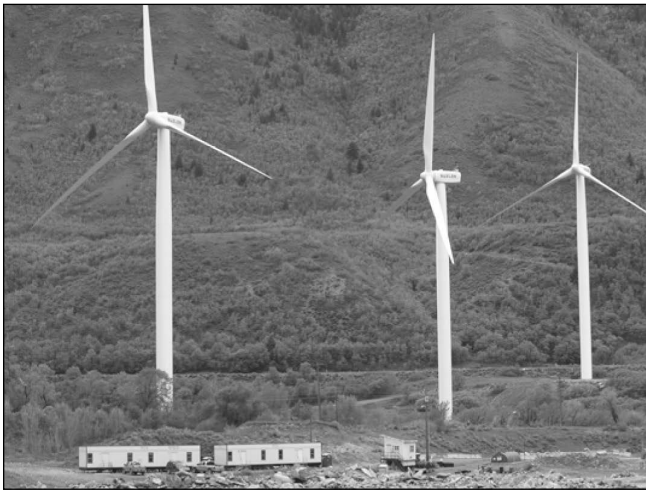
These giant turbines are located in Spanish Fork, Utah. The length of a single blade is 147 feet, and a single turbine is rated to 2.1 megawatts.
