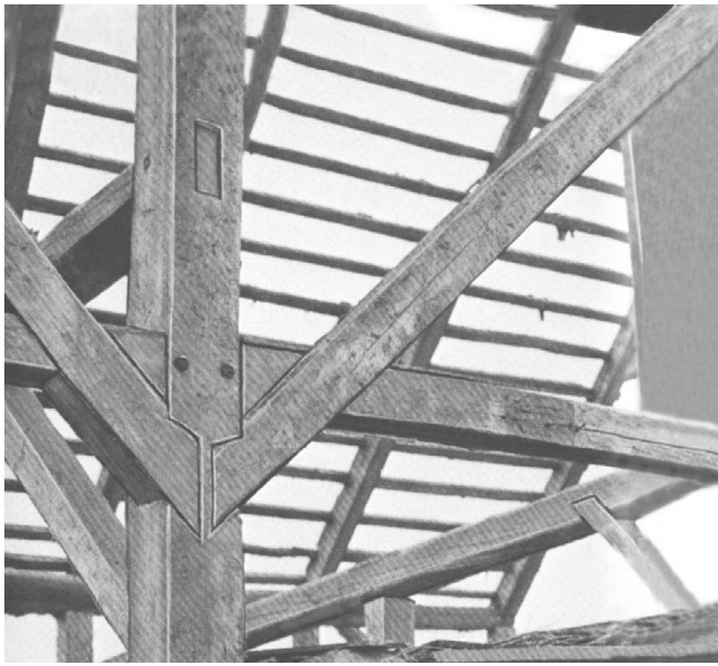
Wooden pegs and well-made joints hold frame of barn together.
