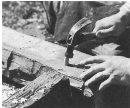
2. Bents are assembled on raising day. Pre-notched, numbered timbers are first pegged together, then braces are cut and fitted.
