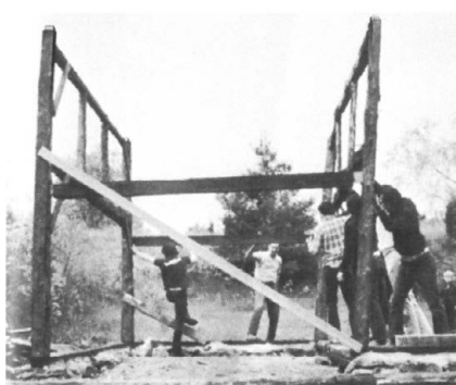
5. The first bent propped, a second bent is raised while several people guide the fitting of the horizontal beams between.
