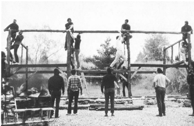
Hoisting each of the top plate beams is a two-stage task. First a beam is raised to crew members stationed partway up; they in turn raise the beam to a group on top.
