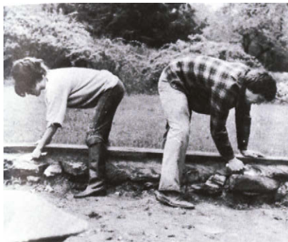
1. Preservative-treated sills, already in place, are mortared to a fieldstone foundation wall. Base of wall must be below frost level.
