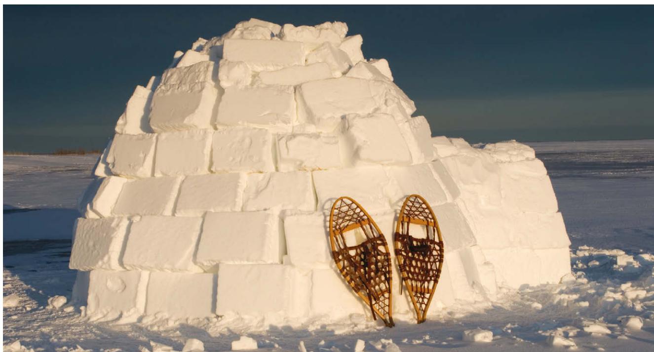
Traditional igloos are constructed from blocks of compact wind-slab snow.
