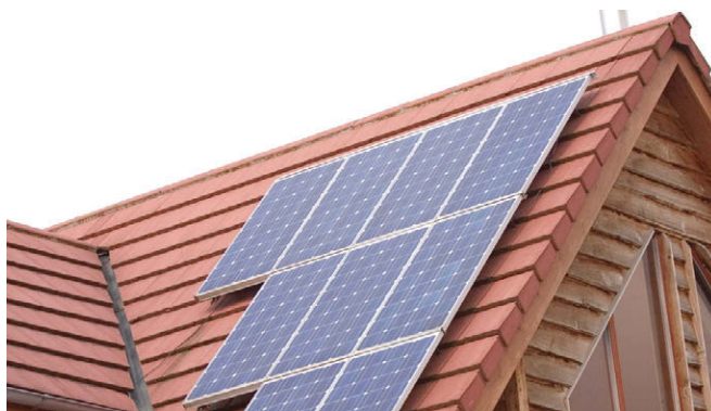
Solar panels on this south-facing roof and large windows on the east side allow the sun to warm the house during the day and provide consistent power. Costs for solar electric cells like these have dropped dramatically the last few decades and continue to become more affordable.
