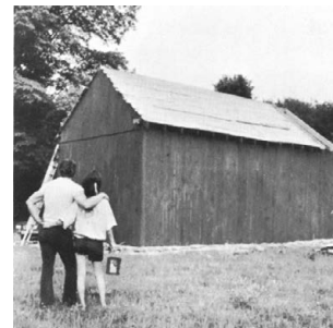
Completing the roof sheathing and putting down shingles are the only jobs remaining. Two coats of barn red give finished structure traditional look.
