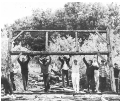
4. Everyone works together to raise the bent into place. Two people check to see that the posts are seated properly.
