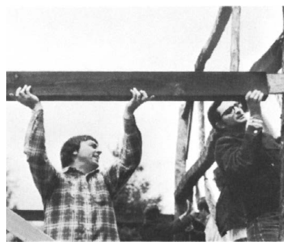
6. Photograph shows how tenons on horizontal beams fit into mortises in posts. Joints will be pegged later.
