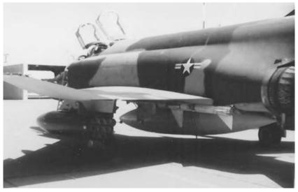
**P-7** View looking forward of the previously described SUU-42 delivery pod. Ejection tubes are clearly visible on the aft portion of the pod. AIM-7 Sparrow missile clearly visible.
